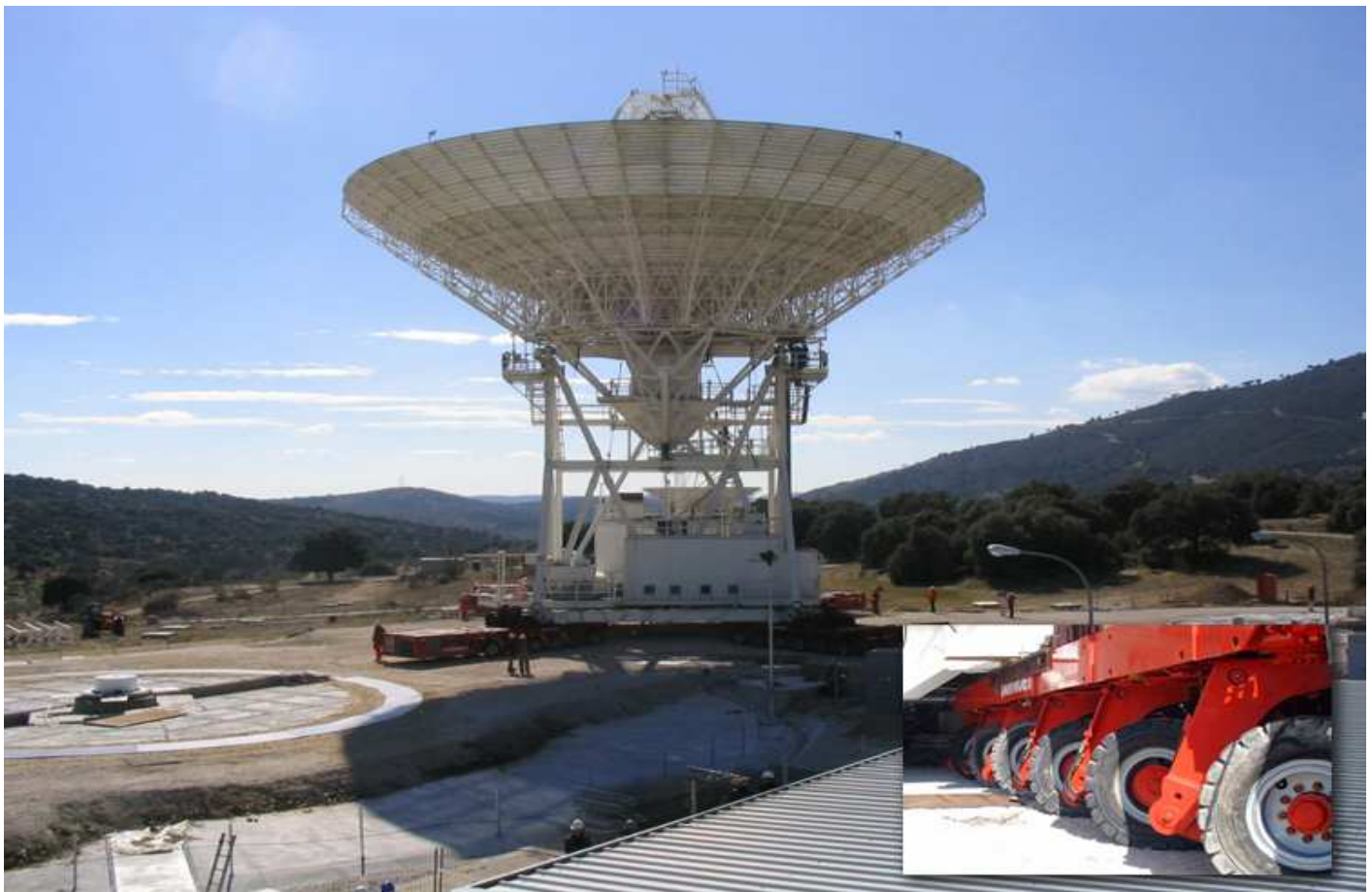
Giant Deep Space Network antenna in Madrid is moved using four 12-axle, 24-wheel crawlers.
